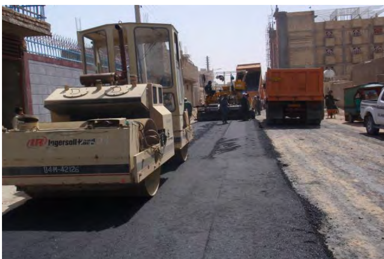
Fig. 18. Construction of a street in Gardez, provincial capital of Paktia in 2012.
