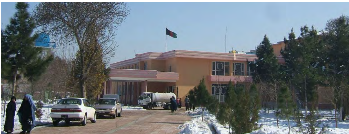
Fig. 8. The building of Mazar-e-Sharif Municipality.
