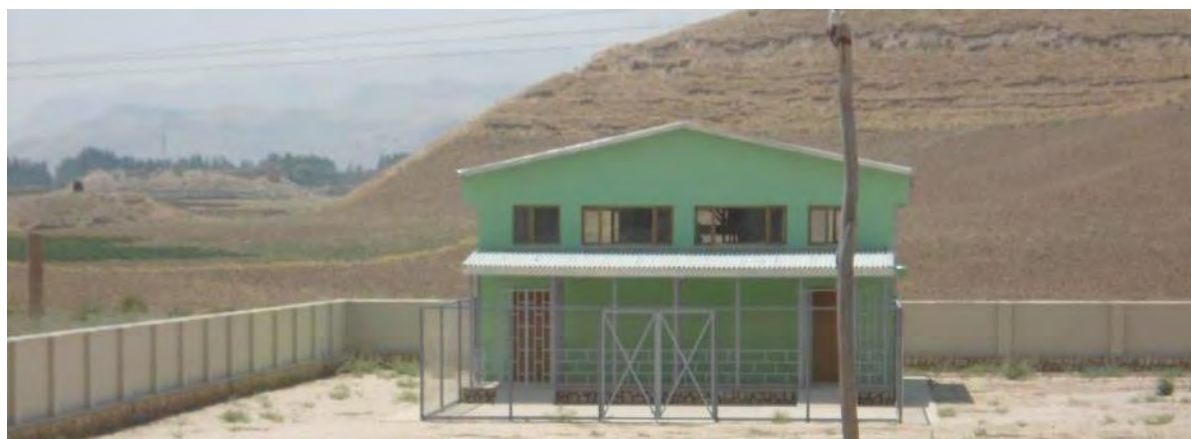
Fig. 15. Municipal slaughter house constructed in Maimana, provincial capital of Faryab province, in 2011.
