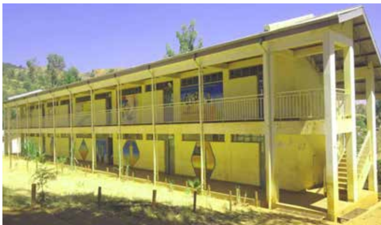
Reji Primary and 2 nd Cycle School built by MIDROC Gold in 2007 E.C
