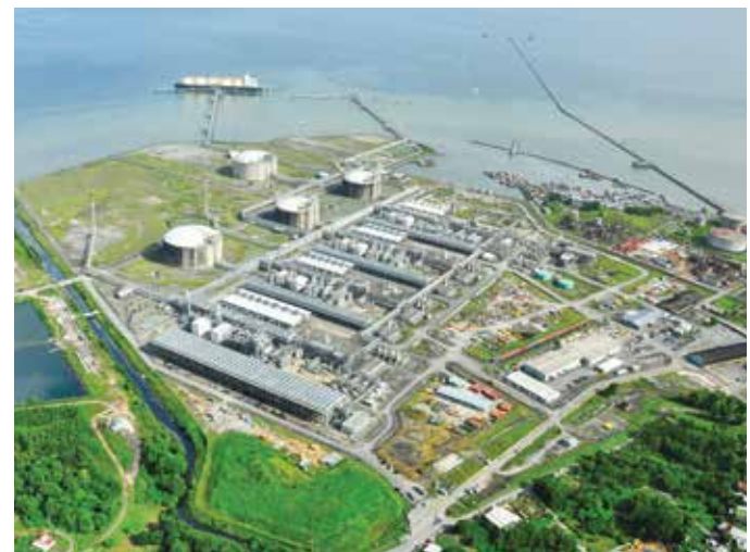
Figure 8: Atlantic's Four LNG Trains at its Point Fortin Facility
