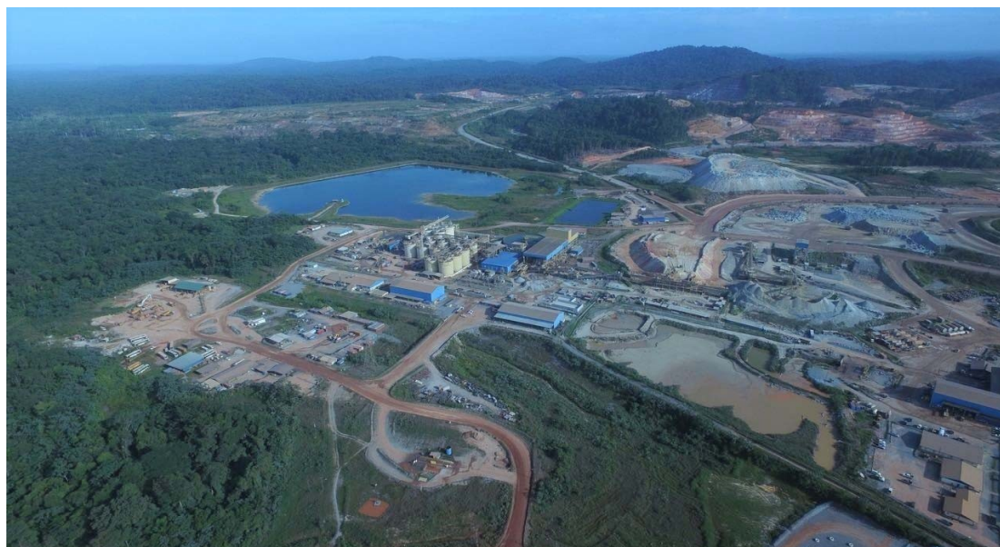
Figure 3.22 Aerial view of the plant of RGM in district Brokopondo, Suriname (source RGM)
